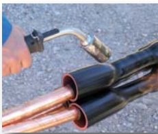
Heatshrink Cable Joints/Splices
