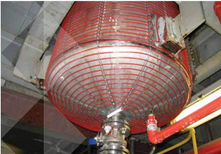
Temperature maintenance of fluid storage vessels with Raychem XPI tracing cable.
