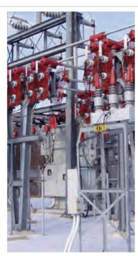
The Raysulate electrical insulation family of products offers easy-to-install busbar insulation systems for both the field engineer and the manufacturer. Raysulate electrical insulation products provide flashover protection against the accidental bridging of conductors commonly caused by birds and animals.
