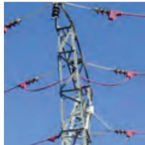
BCIC covers for Dead End connection points and Suspension Clamps protect energised lines from perching, landing and nesting birds.
