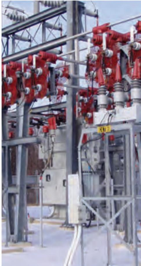
The Raysulate electrical insulation family of products offers easy-to-install busbar insulation systems for both the field engineer and the manufacturer. Raysulate electrical insulation products provide flashover protection against the accidental bridging of conductors commonly caused by birds and animals.
