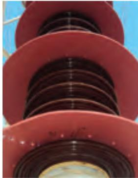
The Booster Shed is a loose fitting collar made from Raysulate anti-tracking polymer which is spaced from the porcelain skirt by short pegs and from the insulator core by spacers. Booster sheds prevent "heavy wetting" flashover by breaking up the water cascades from skirt to skirt. Booster sheds have also been proven to prevent ice-cascade-induced flashovers.
